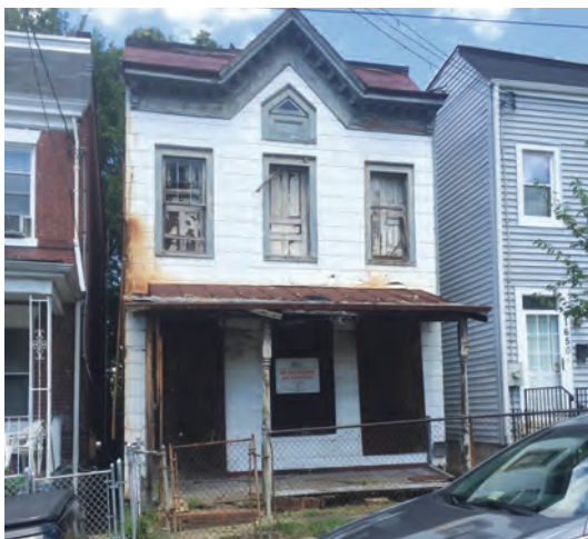
A rusted, stained District house at 1648 U St. SE on the proposed legislation to transfer to L’Enfant Trust.
